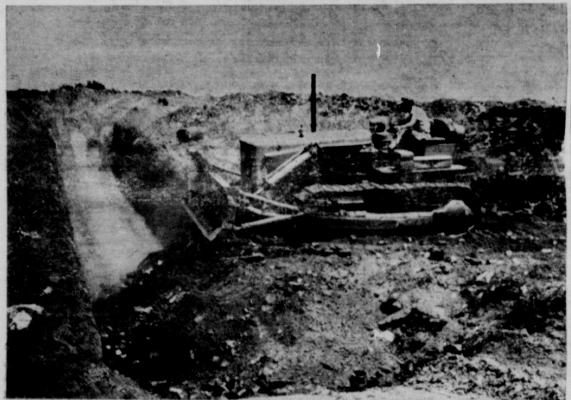
INTO THE PIT: Bob Glenn uses a Gray County bulldozer to push tons of refuse into a newly dug sanitation landfill pit at the McLean dump grounds. The huge pits were dug recently as the City of McLean began the landfill method of disposing of garbage and other refuse. (McLean News Photo)
