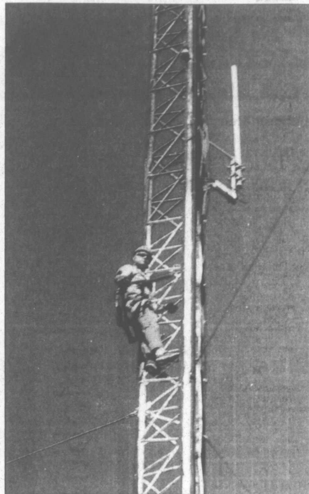
Centramedia's new towers mean an extended service area.
