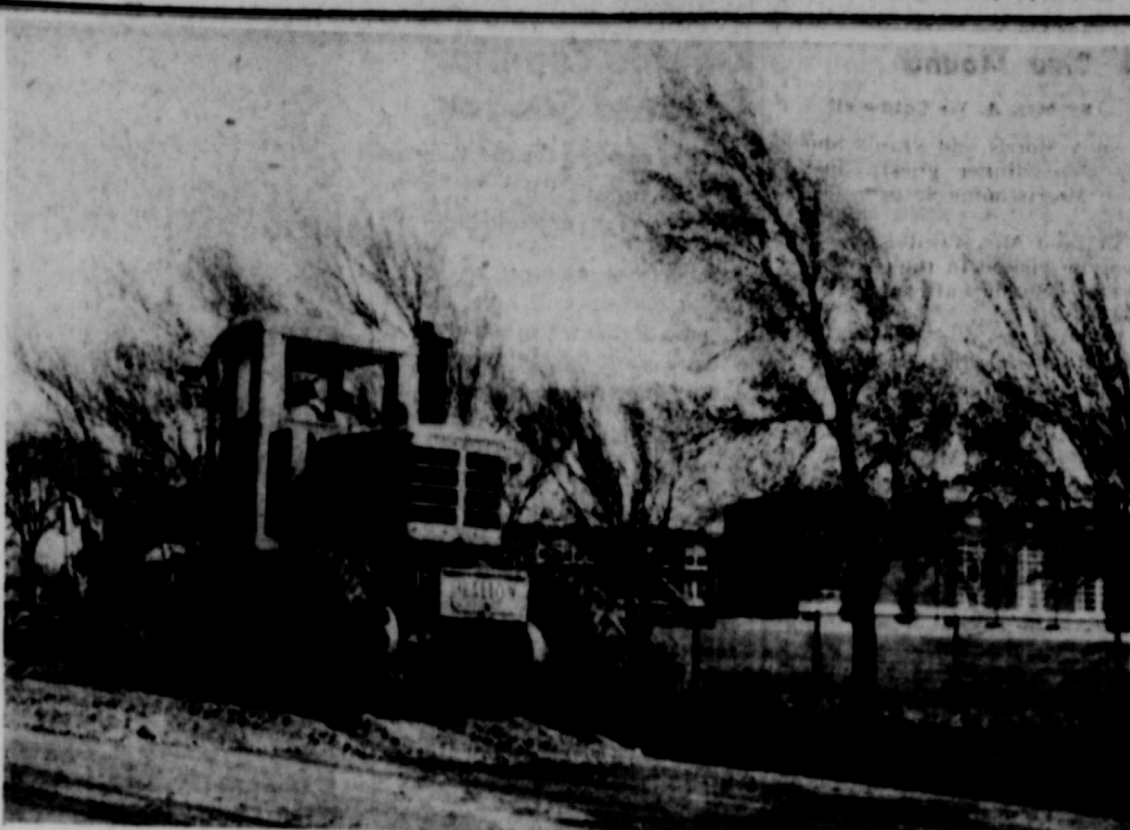
WIDER HIGHWAY —This grader of the Texas Hiway Department is shown at work on highway 117, in west Perryton, which is being widened six feet on both sides this week by the Texas Highway Department. The entire highway to the city limits will be resurfaced within the next few weeks.
