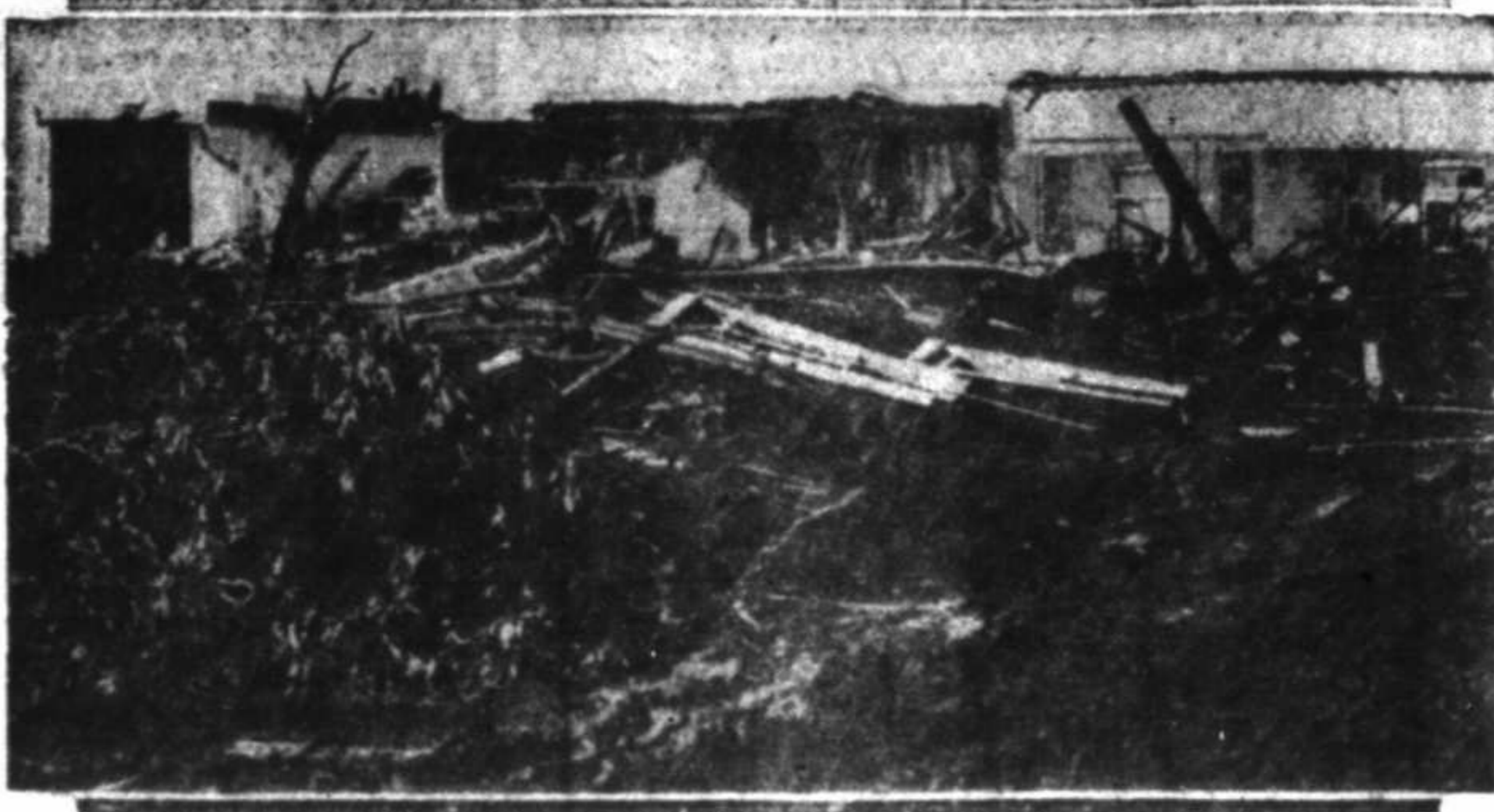
The town of Froot, Texas, was the scene of a terrific tornado which destroyed or damaged every building in the town. This picture shows ruins of entire block of business buildings.
