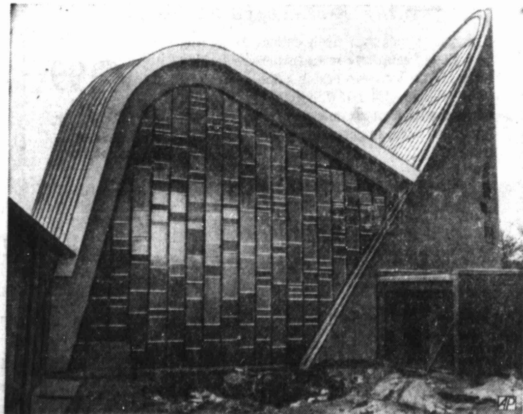
DESIGN FOR WORSHIP — "The Chair of the Lord" is what passersby call this Protestant church under construction in suburban Bremen, Germany. Sides and portion of the top of the concrete edifice are partially-painted panes of thick glass.
