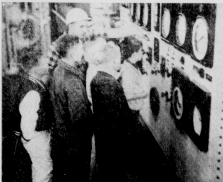
THE OPERATIONS OF the turbine control panel at Tucos are explained by Maurice Tow, Tucos employee, as a group of local seventh graders look on. The photo was made during National Electrical Week when three groups of local seventh graders toured the plant facilities. Groups of students from Petersburg and New Deal Schools visited the plant during the following two weeks.
