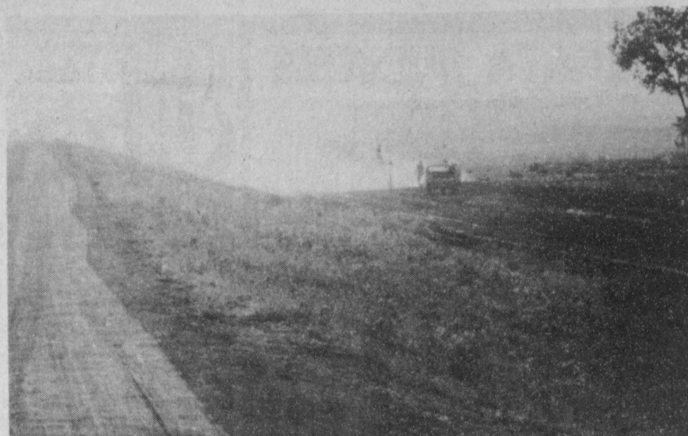
EARLY Morning Fire—The burrs at the base of the Tom Jeffus Reservoir
