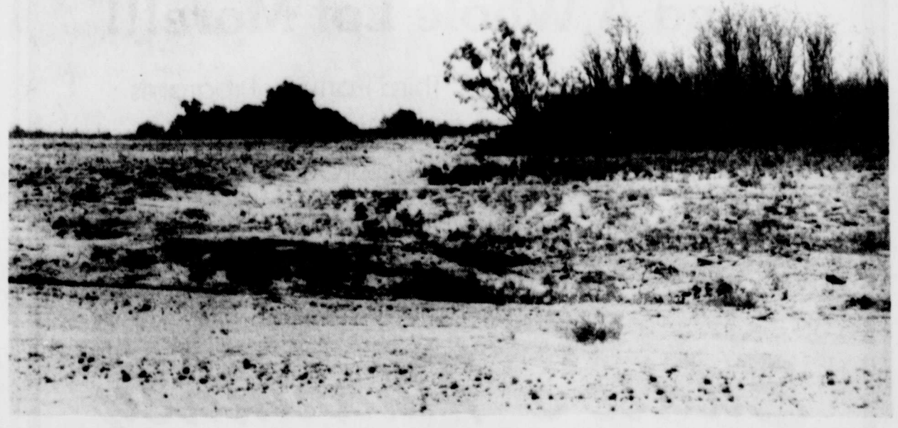
THE SANDLOT AT COLORADO CITY: Work has slowed down at the site where a new softball field is being constructed northwest of town as the city is waiting on results from surveyors in order to give the best usage for the 25-plus acres where plans call for at least two fields along with adequate parking to be built. The city had originally explored the idea of drilling a water well but by using city crews to lay a waterline to the site, over $4000 have been saved.
