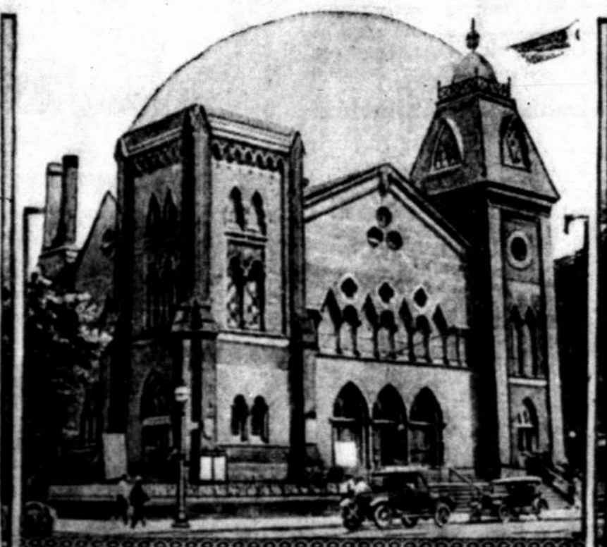
The First Congregational church of Washington, which President Coolidge has attended since he first went to the capitol, has been declared unsafe for public assemblage and ordered permanently closed by the building inspector.
