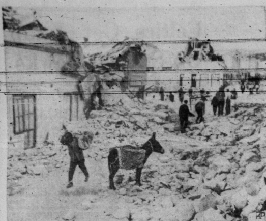
DEATH OF A CITY —Crushed by earthquakes and a tidal wave, the Moroccan city of Agadir is a heap of wrecked buildings and rubble. Survivors salvaged some possessions from homes before the city and its thousands of dead were abandoned.
