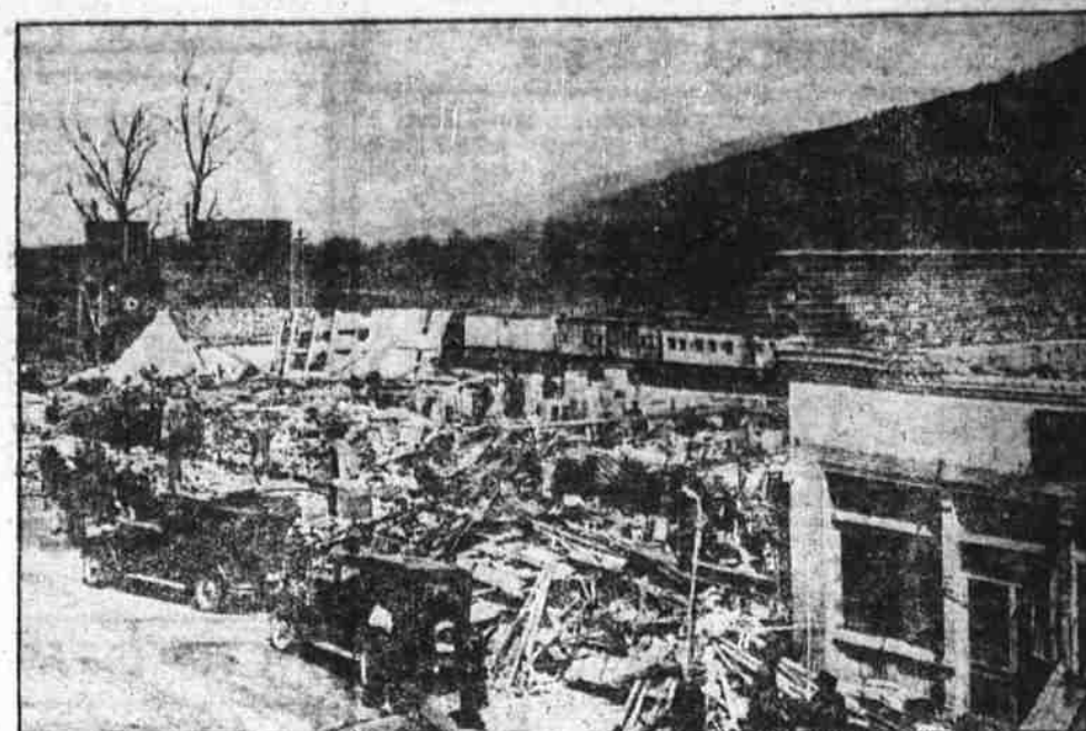
Four persons were killed when a hoistery mill in Paint Rock, Ala., was struck by one of the tornadoes which caused widespread damage and loss of life in the south. The ruins of the mill are shown above.
