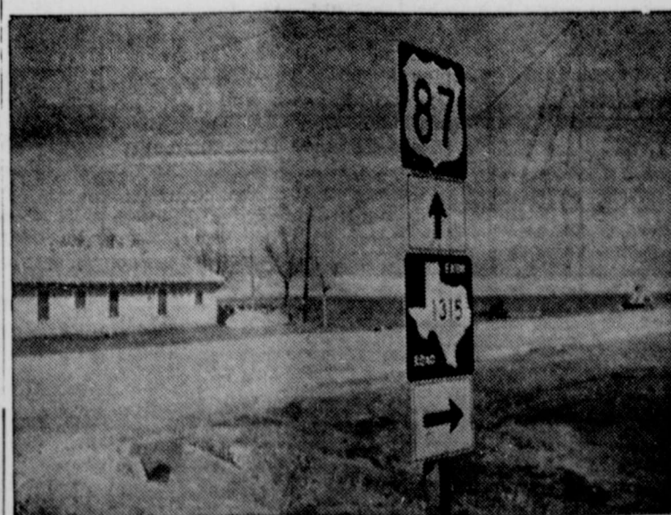
SIGN OF PROGRESS—FM Highway 1315, which comes in from Cotton Center and joins U. S. Highway 87 at the Cotton Boll Gin, now has been paved from Highway 87 east to join FM 400 south of Happy Union. FM 1315 travels U. S. 87 for one mile south of the Cotton Boll Gin to a point ten miles north of Abernathy where the new FM 1315 paving extends east to FM 400.
