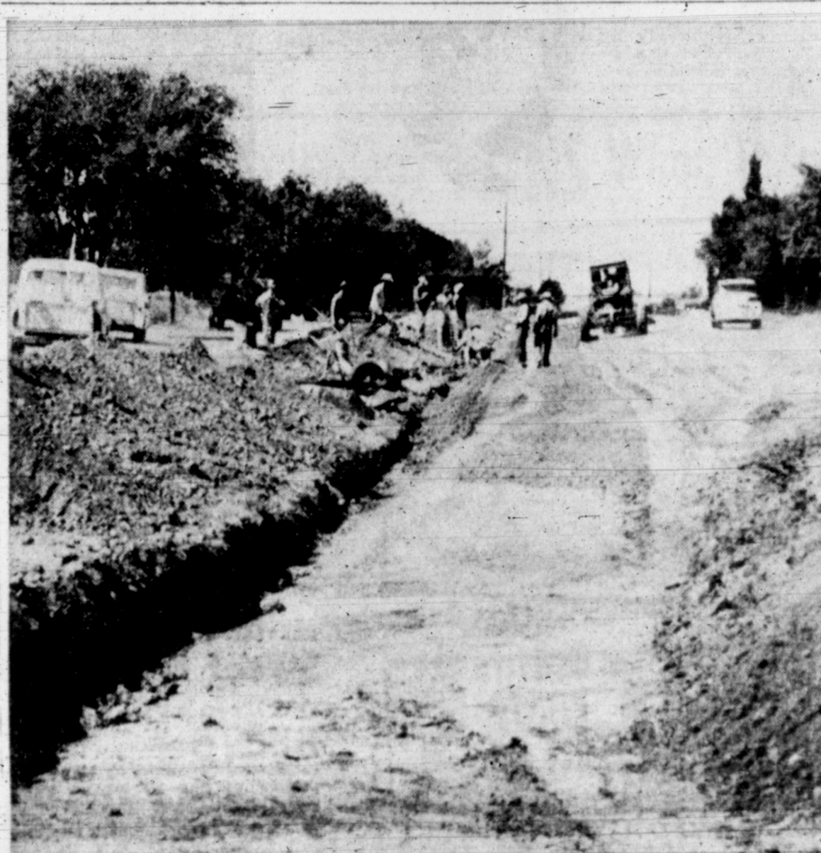
WIDENING DUNCAN STREET
