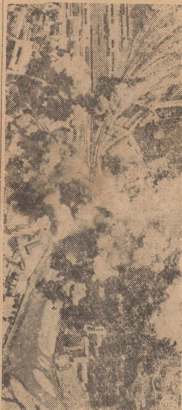
Smoke blossoms mark direct hit on the Bolzano, Italy, railroad bridge near Brenner Pass as Flying Fortresses give another destructive demonstration of their high-altitude precision bombing.
