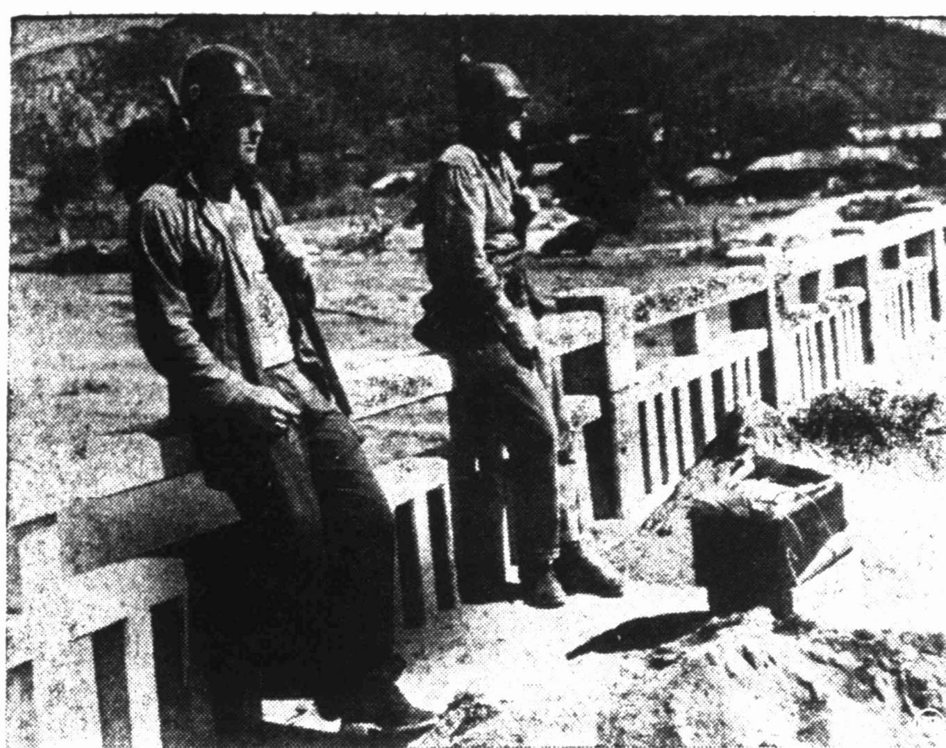
TROOPS GUARD MINED BRIDGE —Pfc. Robert L. Lavdie, Rockaway Beach, Calif., left, and Pvt. G. W. Martin, Fort Worth, Texas, guard a mined bridge near an American 105-mm howitzer position in South Korea.
