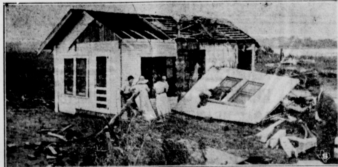
Here is one of a number of farm houses near Brownwood, Texas, that were blown from their foundations by a tornado that recalled the Zephyr disaster in this vicinity several years ago. Three people lost their lives in the recent storm, and a number of others were injured. Damage was extensive in the city of Brownwood, also.
