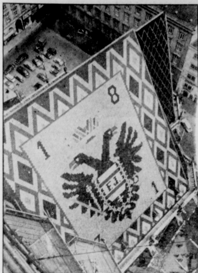
FREEDOM UNDER THE DOUBLE EAGLE —Coat of arms of the onetime dual monarchy of Austria-Hungary and also of the House of Hapsburg once more glitters over an Austria which is once again independent of both royal reign and occupation. Workers have just finished restoring the half-million-piece tile mosaic on the roof of St. Stephen's Tower, Vienna, which was destroyed by fire in 1945.
