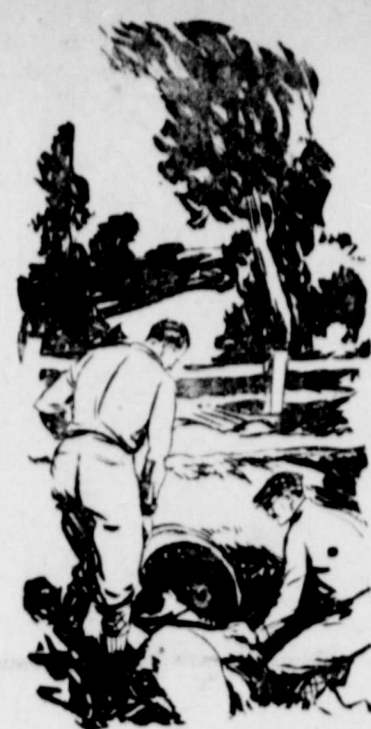
Made an Examination of the Culvert.
