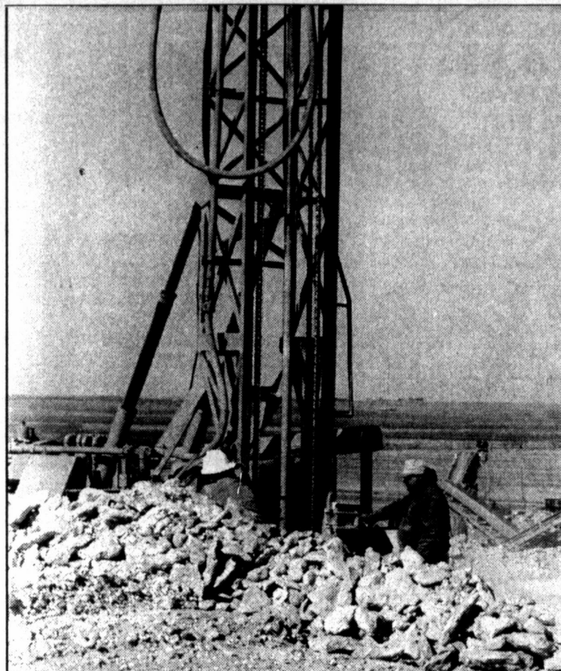
DRILLERS Raul Zavala of Jasper, left, and John Rangel of Colorado City were drilling 20 foot holes in solid rock for dynamite to be placed in at the county rock quarry northeast of Loraine. They work for Lariat Drilling Co.
