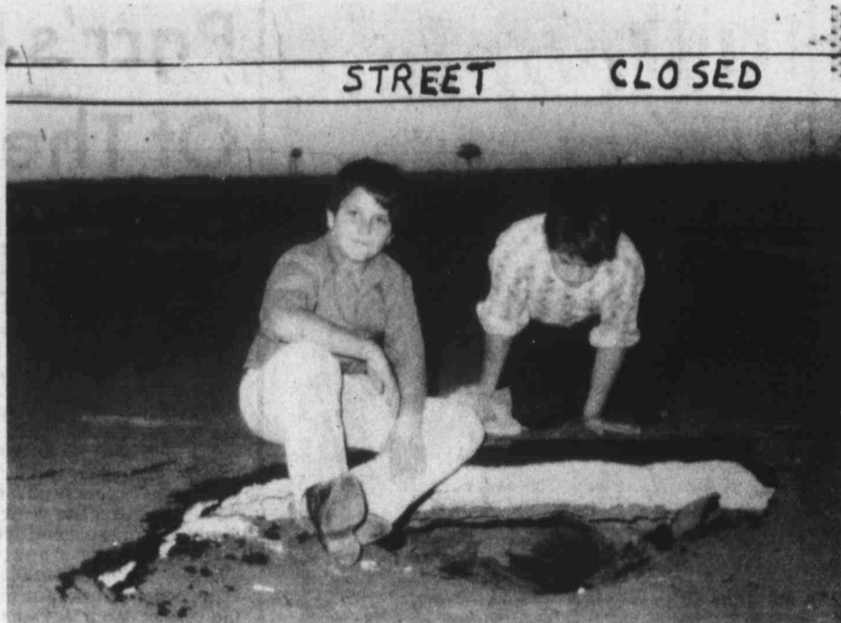
BOTTOM FELL OUT — A newly paved street at 8th and Owens had a big section fall out during the night Tuesday. It is in a location that was once a gravel pit and later filled in before sewer line and street construction. City officials said today that they will dig down to find the cause of the collapse of apparently both the street and sewer line at that location. Bill, 11, left, and Tom, 10, sons of Mr. and Mrs. Glen H. Barber, stop en route home from the YMCA and try to determine the depth of the hole.
