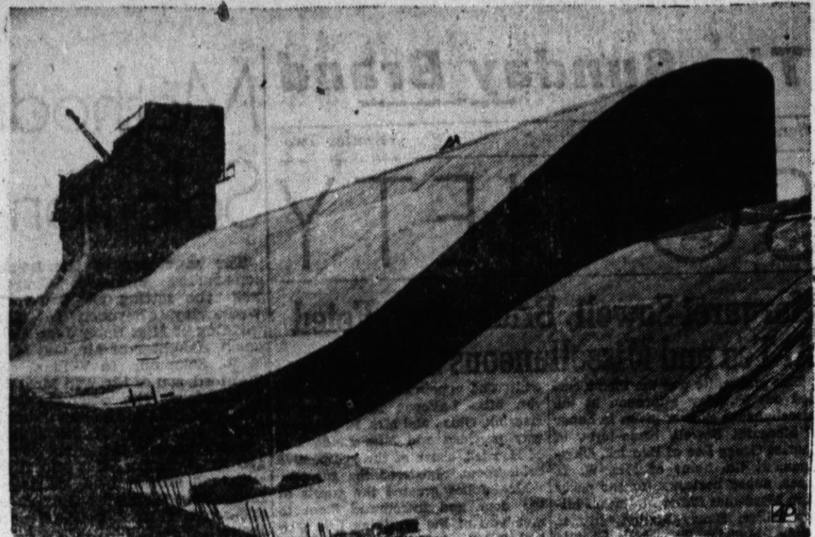
TO HELP CONTROL TRINITY RIVER —This is the partly finished spillway section of the Trinity River's Benbrook Dam. The dam is one of four flood-control projects being constructed along the Trinity River in the Fort Worth area by the Galveston District of the Corps of Engineers. (AP Photo)
