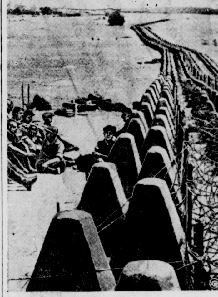
Germany's New 'West Wall'
