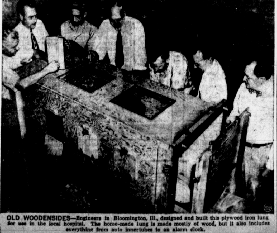
OLD WOODENSIDES—Engineers in Bloomington, Ill., designed and built this plywood iron lung for use in the local hospital. The home-made lung is made mostly of wood, but it also includes everything from auto innertubes to an alarm clock.
