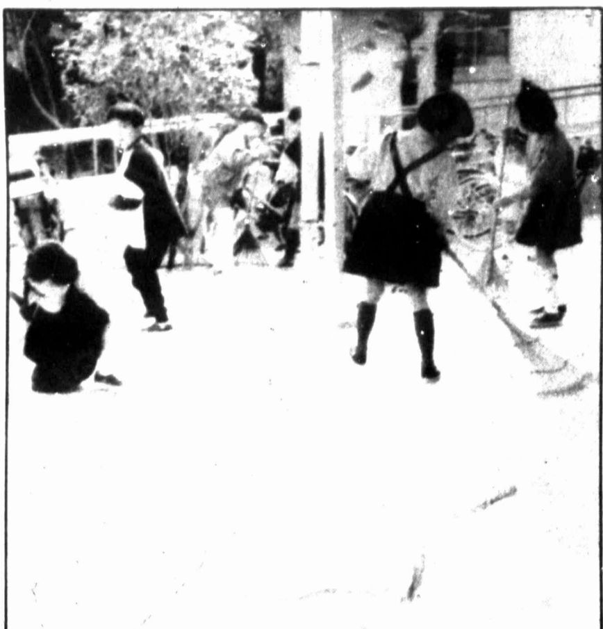
With a crack in the concrete stairs, children sweep the floor at the Muko Elementary School in Amagasaki, near Kobe, western Japan, as the school resumed classes today for the first time since Tuesday's earthquake which claimed more than 4,100 people.
