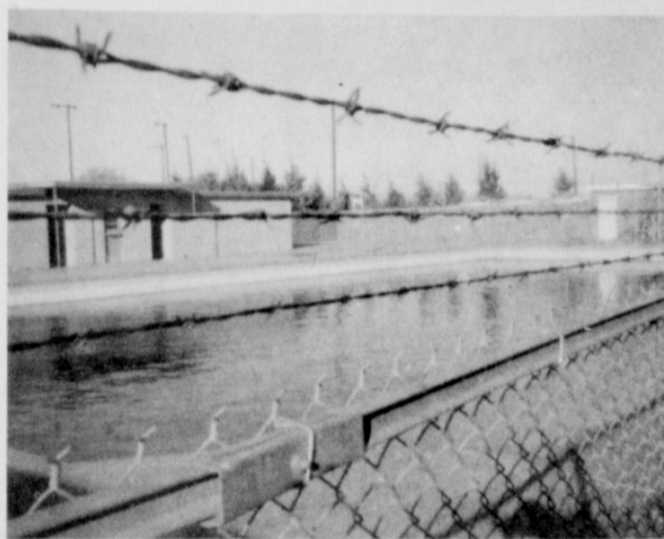
THE TROUBLED WATERS--Pictured above is Slaton's Municipal Swimming Pool, the subject of a complicated controversy this week that raged in Slaton. Trouble began when the U. S. Department of Labor ordered Slaton officials to integrate the pool or be blacklisted for bracero farm labor.
