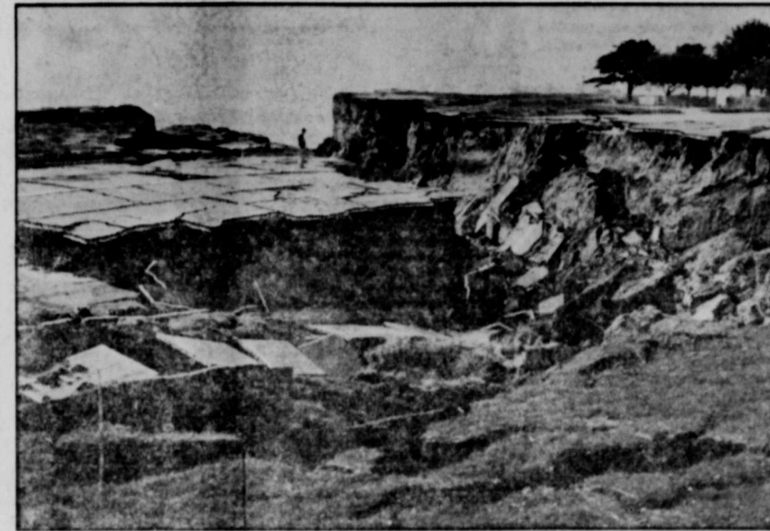
Mahomet may be calling, for the famous shifting mountain at Point Firmin, near Los Angeles, is on the move again. Heavy rains and pounding ocean ground swells caused new sinking of the ground, widening the large cracks in the earth and further breaking up ruined highway on the ocean bluff.
