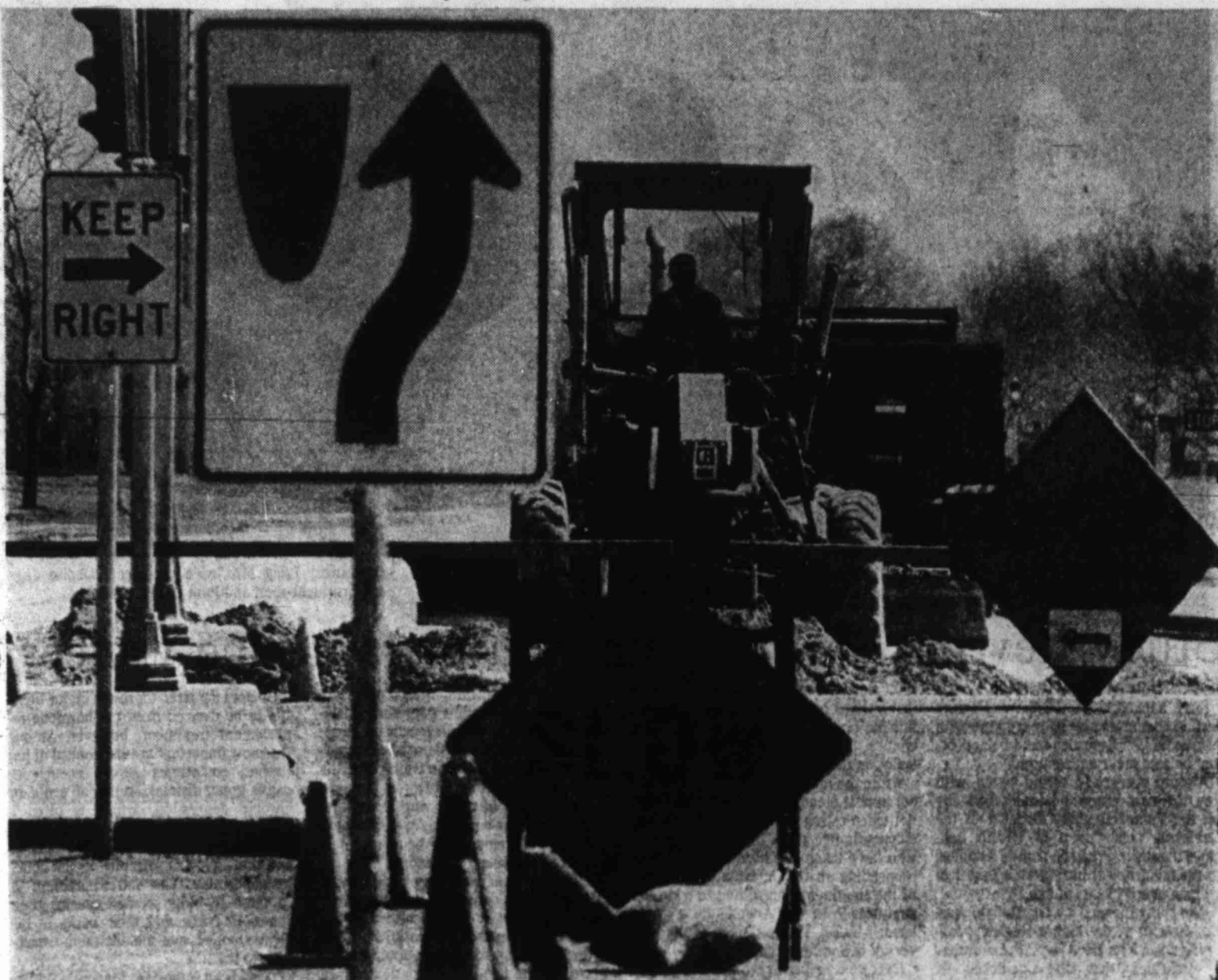
FOLLOW THE SIGNS — Texas Tech's spring break has given city and state road crews the opportunity to repair and resurface Flint Avenue in front of the Tech Agriculture Building, and the myriad signs in the work area could give headaches to anyone trying to drive through. (Staff Photo by Paul Moseley)
