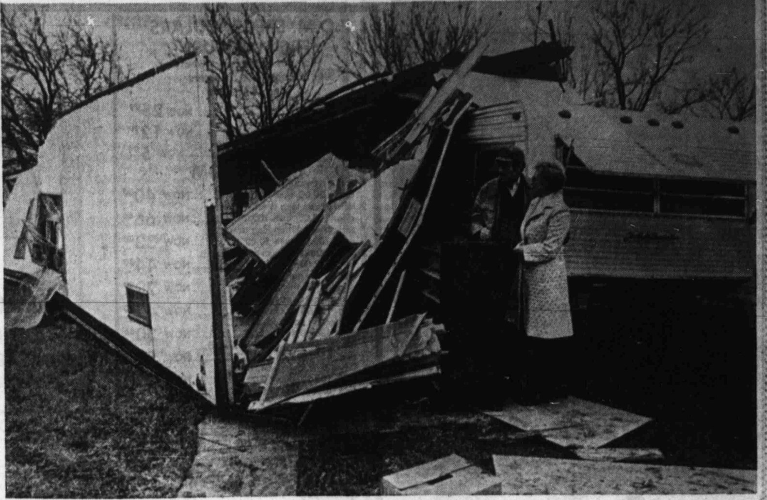
DAMAGE DONE BY HIGH WINDS — John and Judy Recknagel look at the wreckage of a trailer in Plano which was blown over during a thunderstorm accompanied by
