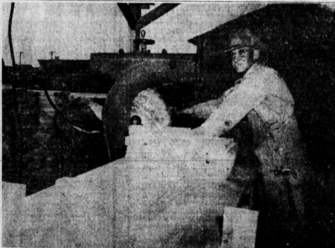
AT WORK ON THE NEW DIMMITT GRADE SCHOOL AND GYMNASIUM on which construction started recently is A. T. Kirby, Dimmitt carpenter who has been in the business about 20 years. Kirby has been a Dimmitt resident for the past eight years. A $375,000 bond issue was voted on July 1 for the building; however bids on the building exceeded available building funds.—Brand Staff Photo.
