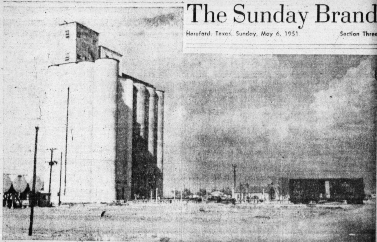
THE DIMMITT WHEAT GROWERS ASSOCIATION is doubling capacity of its elevators at Dimmitt. As shown in the photo, the new bins are being built in the space between the present bins and the boxcar at right. At the time the photo was made, workmen were getting ready for the pouring of concrete which began a few days ago.—Brand Staff Photo.
