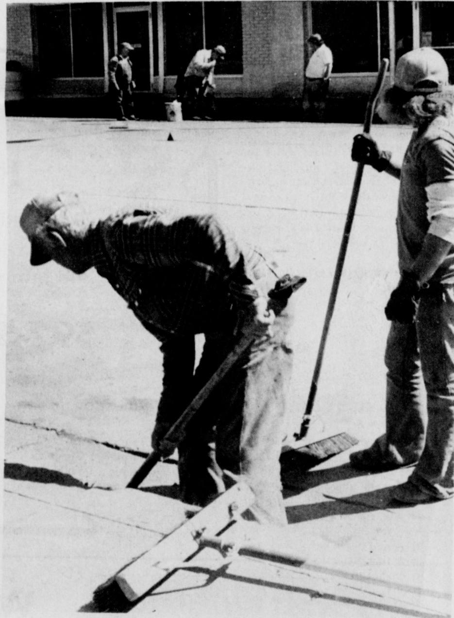
CITY CREW HARD AT WORK ON CASH STREET ... changing angle of parking at curbs.
