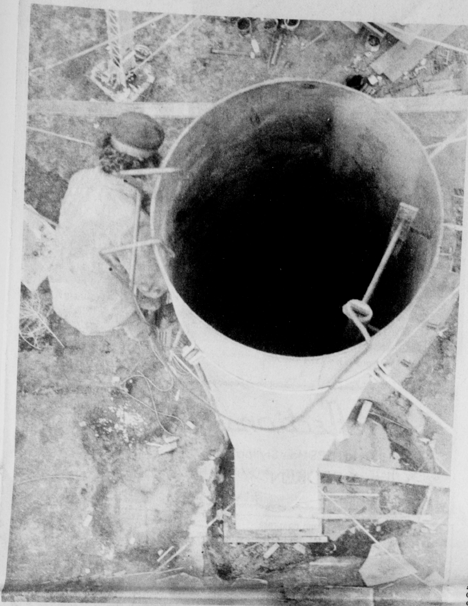
A BIRD'S-EYE VIEW of the construction of Holliday's new water tower was achieved when Lantis Cornutt, operator of the giant crane being used, lifted Leader reporter, Kevin
