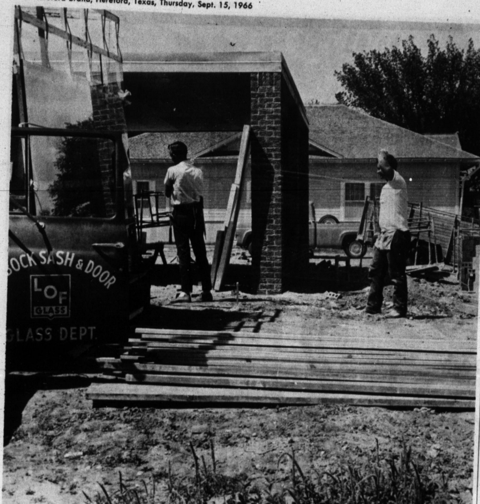
HEAVY AIR? — No, these two workmen from Lubbock Sash and Door are delivering glass windows to be installed in the new Edwards Prescription Pharmacy building at the
