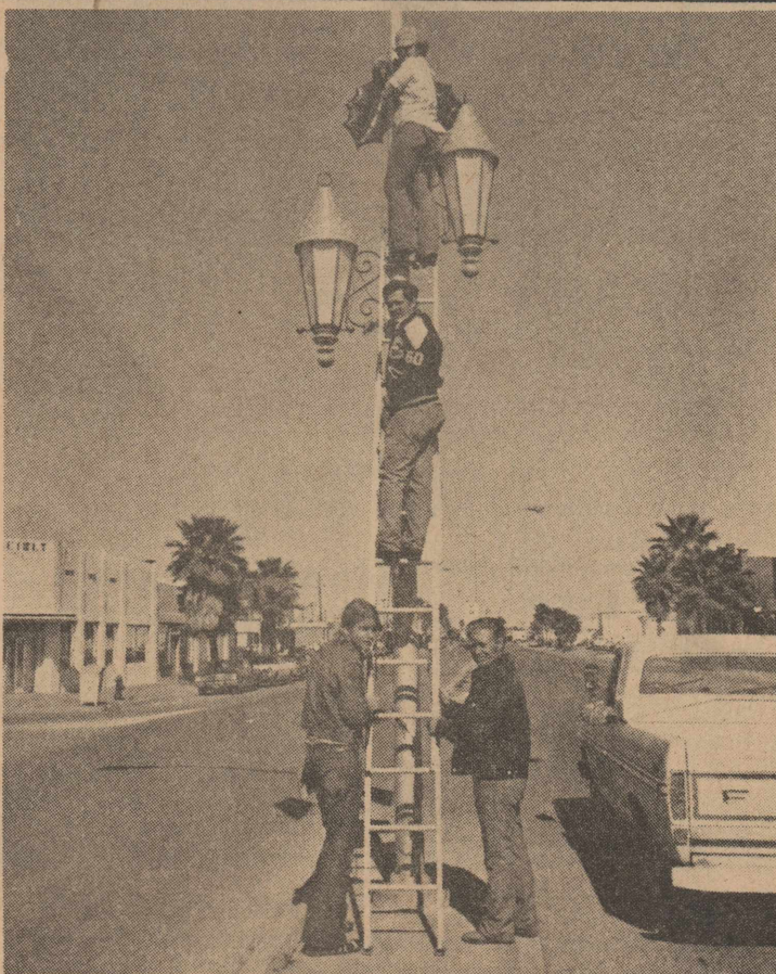
George Miller (lower right) and his business associates, (top to bottom) George Miller, Jr., Charley Cady, Jr., and Jeff Jeffries, installed Christmas street decorations in Rockport and Fulton last weekend, volunteering their services.
