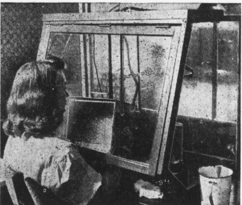
As in every other step of the preparation of sera, vaccines and anti-toxins, extraordinary precautions are taken in bottling the products. A glass window covers most of the filling operation to prevent air contamination.
