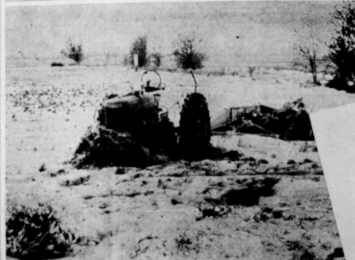
FLOOD DAMAGE—Rushing flood waters during the first part of last week did considerable damage to farms and equipment all over the western part of the county. An example of this is the tractor and land leveling machine above which was washed for about 200 yards from the T. H. Gattis farm over a field farmer by Son Hunter. Most of the damage was inflicted in the area where farmers are trying to get a series of dams constructed on the headwaters of four creeks.
