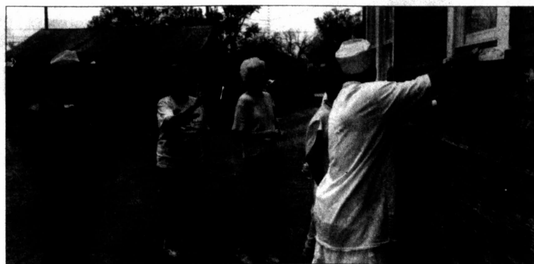
CHRISTMAS IN ACTION'S Joyce Robertson (second from left) and Georgie Griffith (center) instruct TDCJ workers in the fine art of scraping paint from the exterior of a house during prep work for next week's CIA community-wide rehabilitation effort. TDCJ guard Willie Davila looks on.
