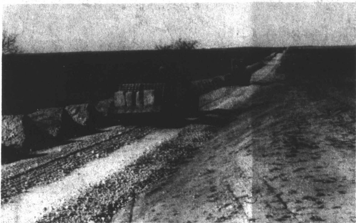
ROAD WORK: County employees are shown using the equipment which grades, background, and the grid-roller, foreground, to crush the mounds of road material which has been stationed at the section of county road 464, in eastern Mitchell County, that is currently being repaired.
