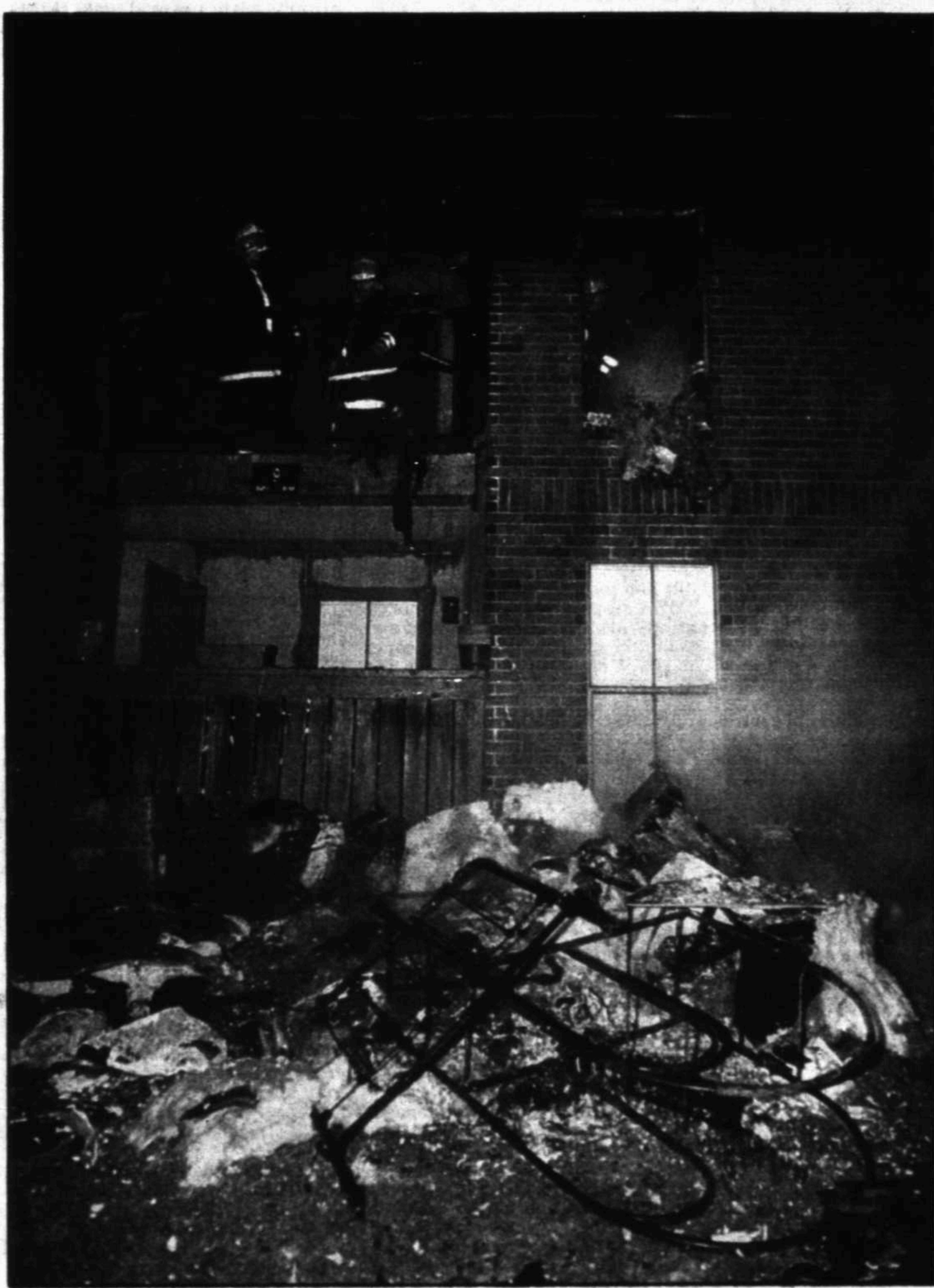
Midland firefighters stand in a second-floor apartment gutted by fire late Tuesday. No injuries were reported in the blaze at the
