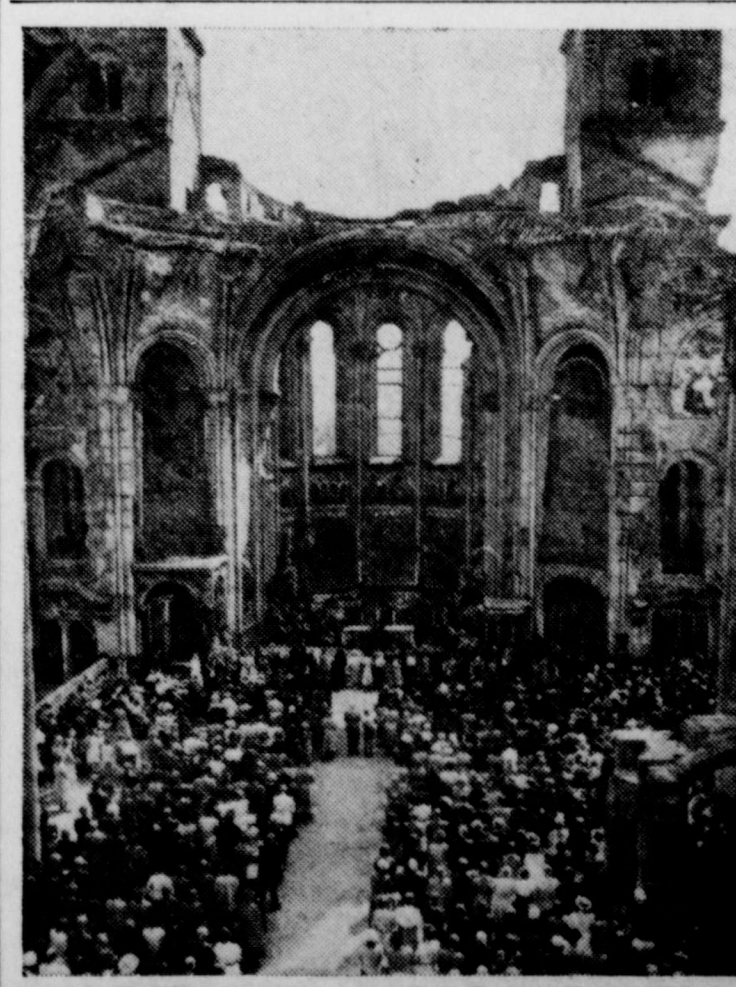
STILL IN USE—Worshippers in West Berlin's Kaiser Wilhelm Memorial Church ignore the roofless condition of the city's famed landmark and crowd into church services in the bombed-out structure. It isn't too bad on bright, summer days.
