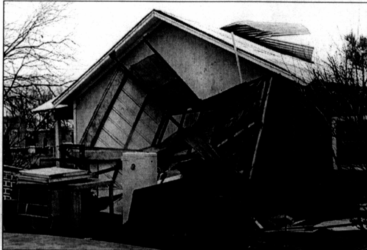
A STORAGE BUILDING WAS RIPPED from its foundation and thrown against an adjacent house on Pacific Street in Loraine by a weak tornado produced by a fast-moving thunderstorm that roared through Mitchell County on Thursday, March 4. The storm also damaged the home's tin roof. The tornado uprooted large trees and knocked out power to 20 to 30 homes, according to Randy Ward of Oncor.
