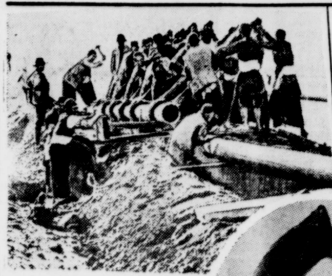
Iraq Forces Reported Seizing Oil Fields — Iraq—Laying pipeline carrying the rich oil of Iraq to ports on the Mediterranean.
