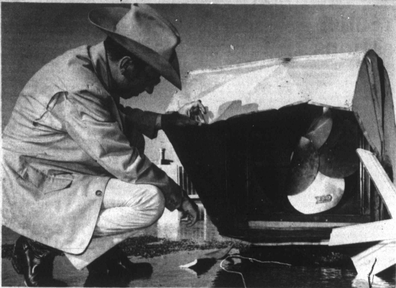
A SMALL CULPRIT? — Ken Kieth examines a circulating fan and duct which were damaged during a break-in at the Harvester Lanes bowling alley on Highway 70 early today. The burglars, apparently frightened away when a janitor came to work at 4 a.m., dropped three
