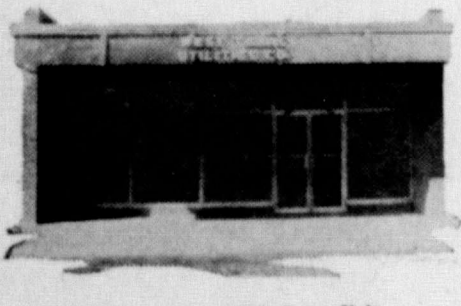
Recently remodeled WTU office at Clyde
