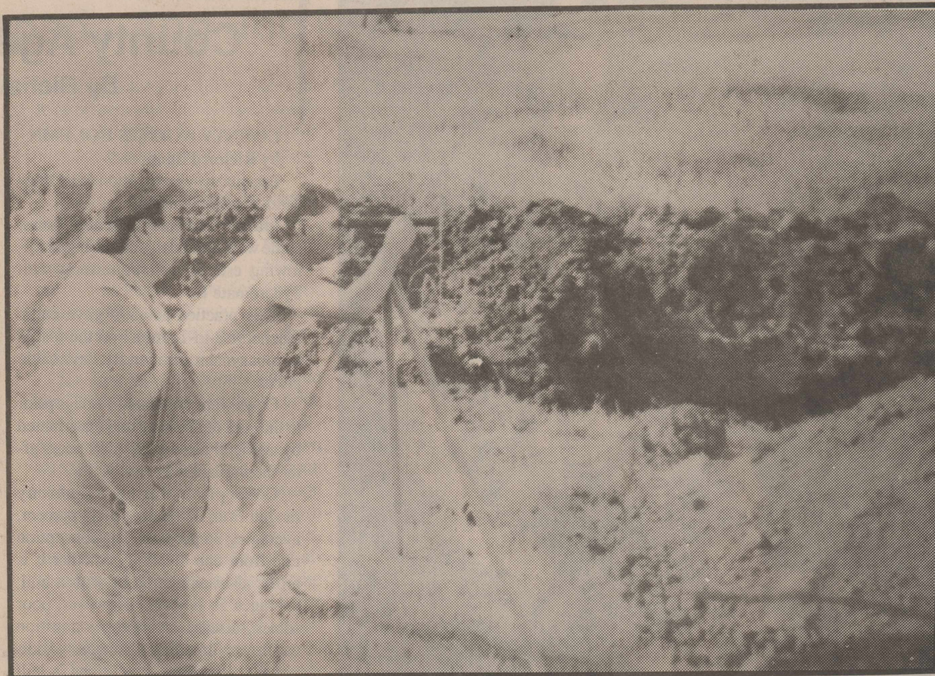
INSTALLING DRAIN PIPE: Two City of Rotan employees, Randy Martin, left, and Rodney Denton, Jr., right, survey the slope of the land near the swimming pool and golf course. The city crew is in the process of installing a new drain pipe from the swimming pool east.
