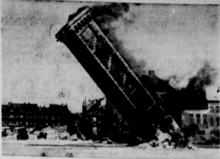
FALLING TOWER . . . Tower of old station in Ostend, Belgium, is blasted to make way for exposition scheduled for 1958.
