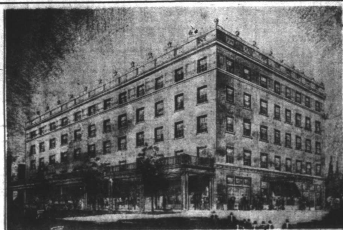
New $350,000 Hotel Grayson Now Under Construction to be Completed Early in 1927.
