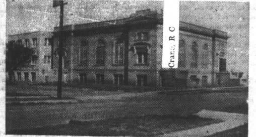
University Church Building, Abilene, Texas.
