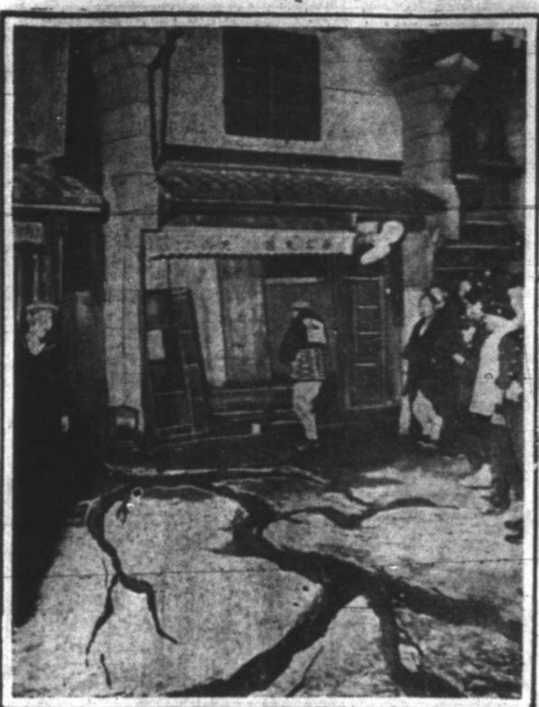
A temblor which rocked the central part of Japan on March 7, demolished several towns and claimed more than 2000 lives. This picture, taken at Osaka, shows the great cracks rent in the earth by the quake. It clearly shows how difficult it is to construct buildings that will withstand Japanese quakes.
