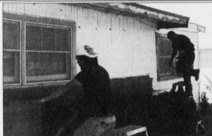
FOUR SEASONS WORKERS add insulation to a Christmas in Action home project early this month. Photo courtesy of Jan Lemons.
