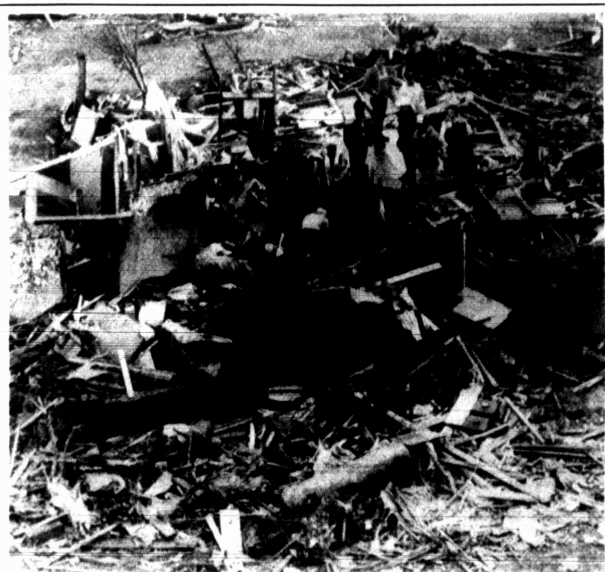
Saragosa residents and family and friends pick through the rubble of what was one of many adobe homes destroyed by a tornado May 23. The town's residents now look to rebuilding their homes.
