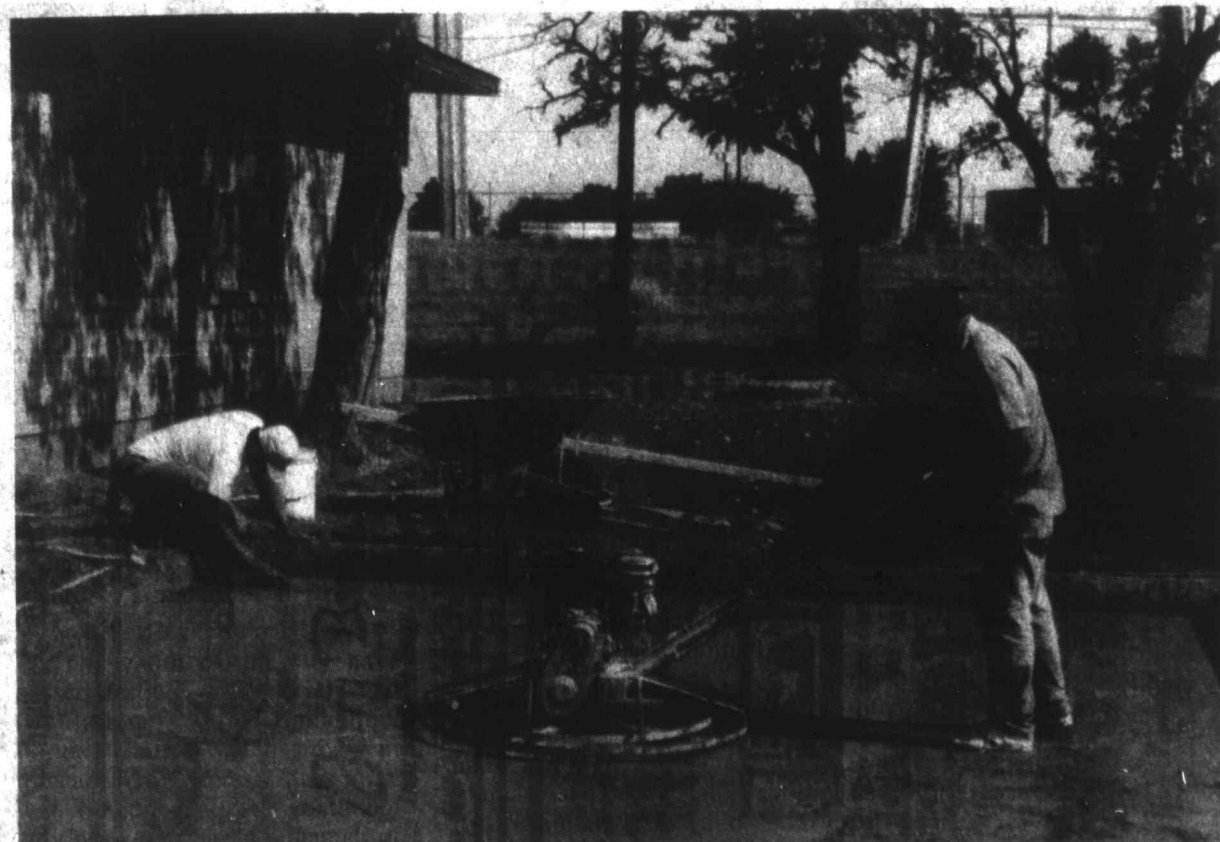
HOUSING AUTHORITY RENOVATIONS: Concrete work to provide a driveway was being done on Tuesday as part of the renovation and remodeling jobs that have been funded for the project homes in the northern portion of Colorado City.
