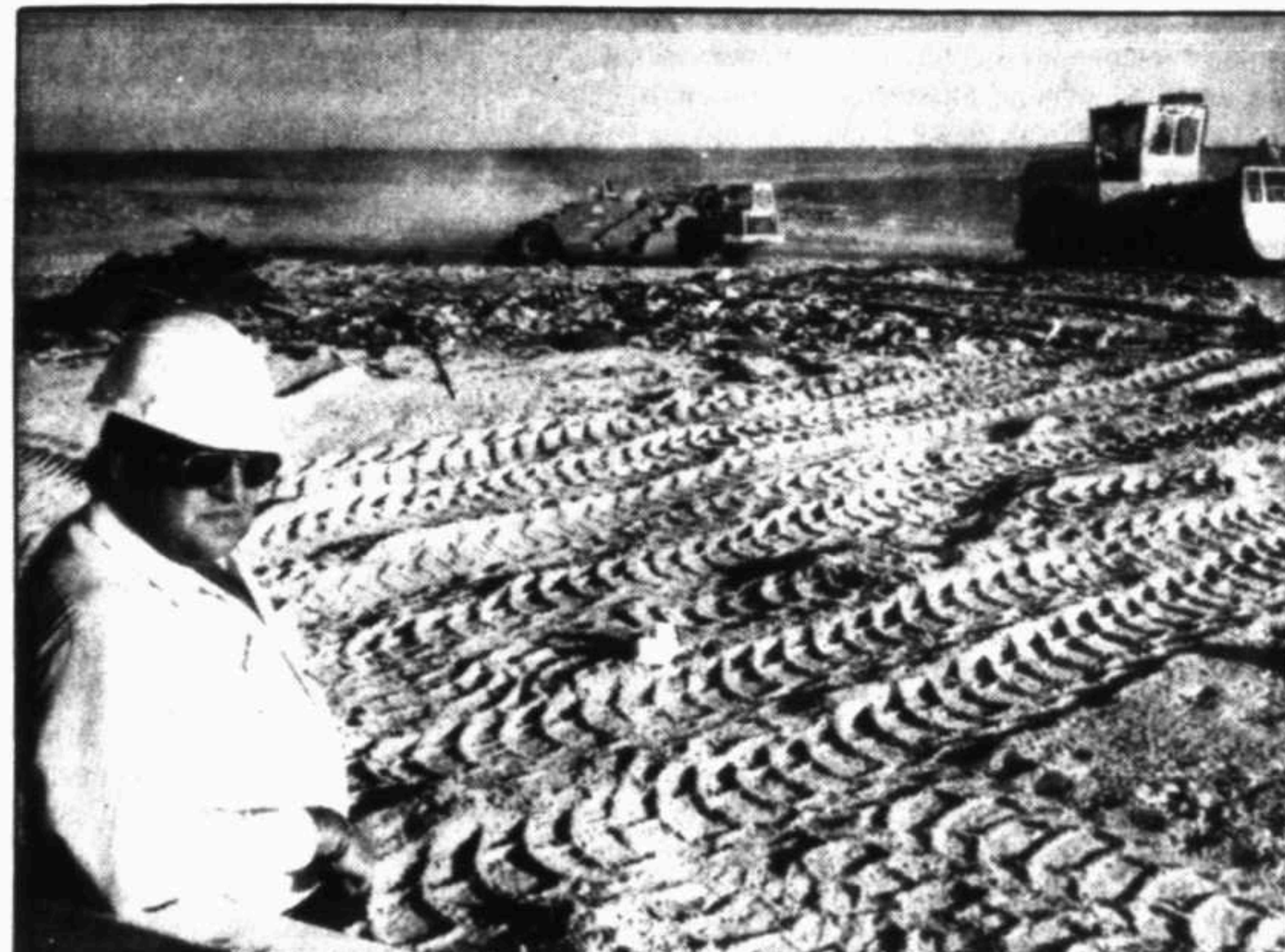
Supervisor Jim Rector checks out work being done at the Midland landfill.
